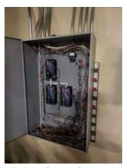
**Photo #146** Reliable Controls field controllers for central plant.
