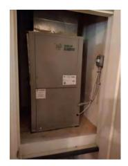
**Photo #119** Older WSHP (vertical orientation) in mechanical closet for dwelling unit.
