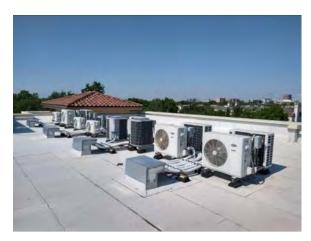
Photo #115 Newer DX split system condensing units.
