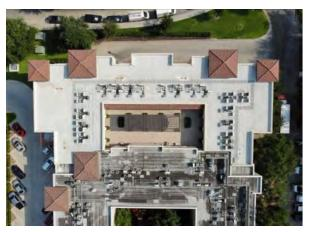
**Photo #30** Overview of modified bitumen roof over the Plaza North Expansion.
