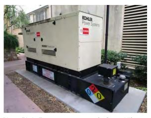
**Photo #152** Emergency generator for fire and life safety systems.
