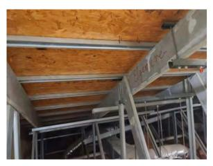
**Photo #22** View of OSB roof deck supported by metal framing.
