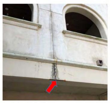
Cracked Facade At Soffit
