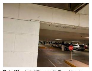
**Photo #58** Joint of Phase II with Phase I in main parking structure showing crack on CMU wall and water damaged. beam.
