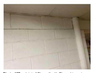
**Photo #57** Joint of Phase II with Phase I in main parking structure showing crack on concrete masonry unit (CMU) wall.
