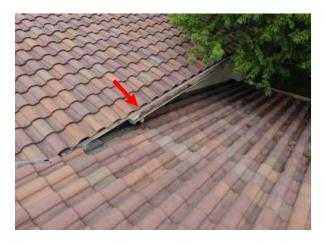
**Photo #27** Typical gutter clogged with debris. Note tree encroachment of roof.
