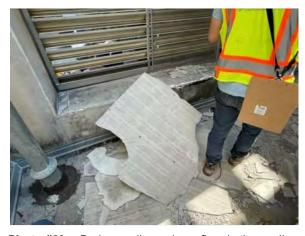
**Photo #63** Broken wall panels on floor in the cooling tower.
