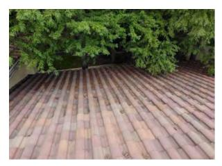
**Photo #26** View of debris build up on roof. Note tree encroachment of roof.
