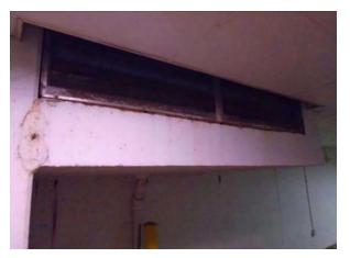
**Photo #162** Outside air intake for parking structure ventilation.
