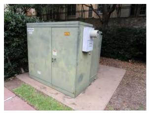
**Photo #149** Typical utility transformer and electric meter for electrical service to the building.
