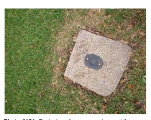
**Photo #154** Typical sanitary sewer clean out for building.
