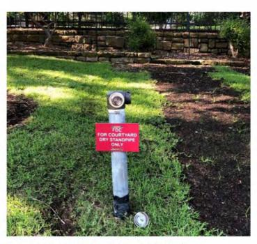
Exterior Post Indicator Valve and Stand Pipe
