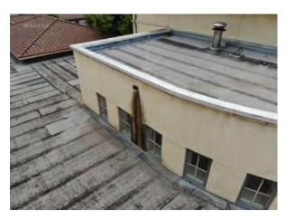
**Photo #46** View of water staining to wall surface from scupper.
