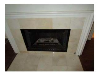
Photo #133 Typical natural gas-fired fire place.
