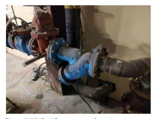
**Photo #105** Backflow preventer for main water distribution.
