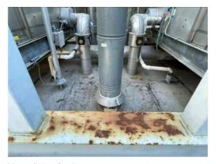
**Photo #62** Cooling tower structure shows deterioration.
