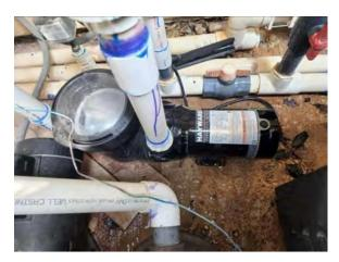
Photo #109 Leaking pool circulation pump.
