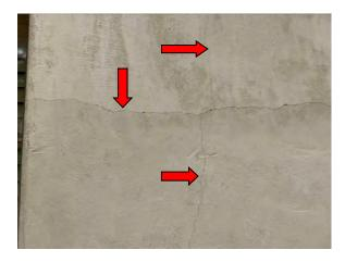
Photo #69 Random cracks in stucco.
