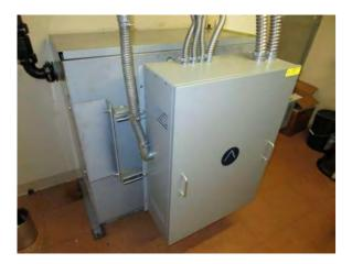
**Photo #136** Typical hydraulic elevator equipment.
