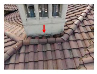
**Photo #44** View of water staining at the base of the chimney.
