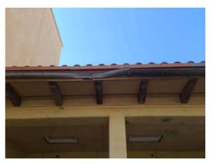
Photo #48 View of severely damaged gutter.
