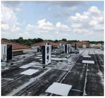
Various Condensers Installed As Replacements
