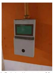
**Photo #160** Typical parking structure CO sensor for ventilation system.
