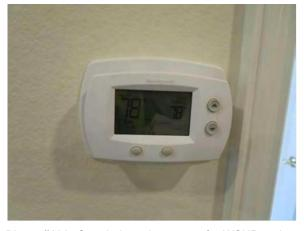
Photo #122 Stand-alone thermostat for WSHP and DX split systems in dwelling units.
