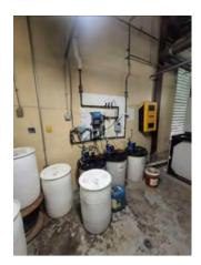
**Photo #103** Automated chemical feed system for cooling tower.
