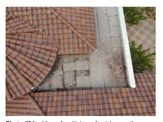
**Photo #34** View of multiple roof patches on the modified bitumen roof.
