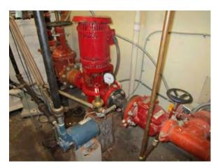
Photo #139 Fire sprinkler suppression pump.
