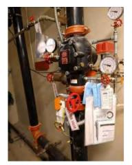
**Photo #138** Dry-type fire suppression riser for parking garage.
