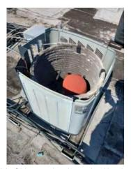
**Photo #114** Older condensing unit with missing condenser fan and motor.
