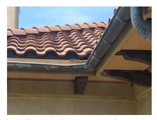
**Photo #47** View of staining on gutters from overflowing water.
