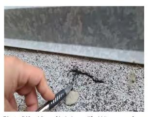
**Photo #40** View of hole in modified bitumen roof membrane base flashing.
