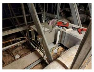
**Photo #112** Ceiling hung water source heat pumps (WSHPs) for dining and other common areas.
