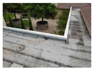
**Photo #35** View of severe loss of granules on modified bitumen roof
