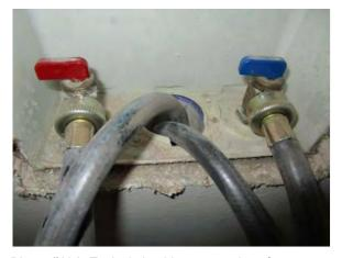
**Photo #134** Typical plumbing connections for dwelling washer.
