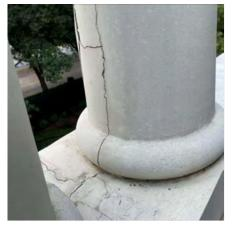
**Photo #72** Isolated crack on exterior architectural column cover in dwelling balcony.
