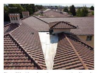
**Photo #28** View of standing seam metal roof in roof valley.
