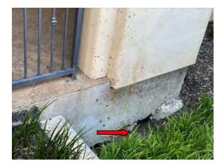
**Photo #71** Scour on the joint of Phase II with Phase I above main basement.
