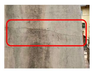
Photo #70 Random cracks in stucco in general.
