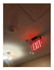
**Photo #148** Path of egress exit sign with smoke detector and fire sprinkler head.
