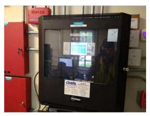
Photo #142 Fire alarm control panel.
