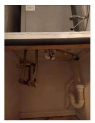
**Photo #120** Condenser water piping and auto balancing valves for WSHP.
