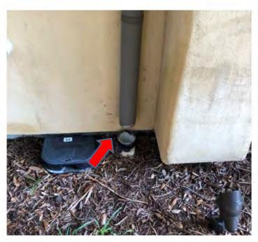
Missing Downspout Connection
