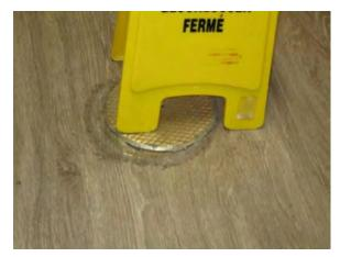
**Photo #155** Loose sanitary clean out cover near kitchen.
