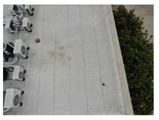
Photo #32 Close view of modified bitumen roof.
