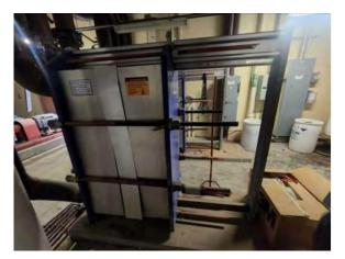
Photo #102 Plate-frame heat exchanger.
