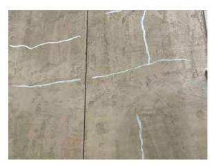
**Photo #67** Repaired cracks in stucco at several locations.
