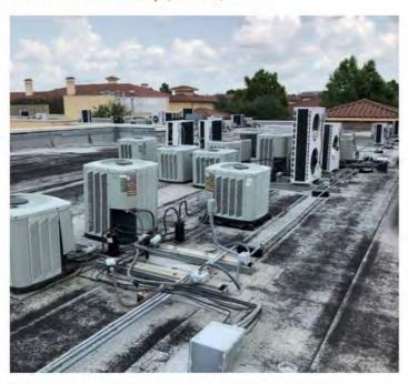
Various Condensers Installed As Replacements
