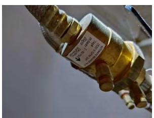
Photo #121 Close-up view of auto balancing valve for WSHP.
