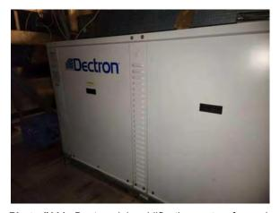
**Photo #111** Dectron dehumidification system for pool area.
