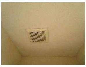
Photo #130 Typical exhaust fan in dwelling bathroom.
