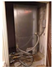
Photo #118 Newer WSHP (vertical orientation) in mechanical closet for dwelling unit.
