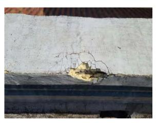
Photo #52 View of damage to EIFS coping.
