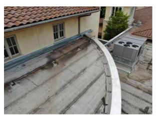
**Photo #38** View of staining on the modified bitumen roof.
