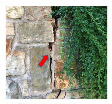
Cracked Mortar Joint in Retaining Wall
