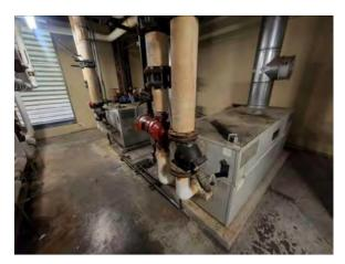
**Photo #97** Auxiliary heating hot water boilers for water source heat pump system.
