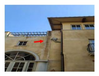
Photo #51 View of staining on stucco façade.
