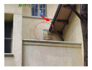
**Photo #49** View of debris clogging downspout and wall repair. Note wall repair and repainting.
