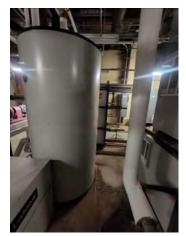
Photo #101 Storage tank for domestic hot water.
