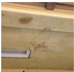
Photo #55 View of staining on ceiling.
