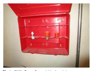
Photo #141 Spare fire sprinkler head storage case.
