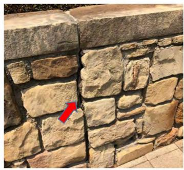
Cracking Tree Planter Due to Expansion
