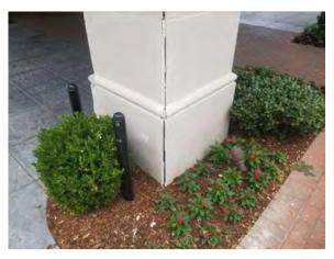
Photo #16 Damaged column at East Porte cochere.
