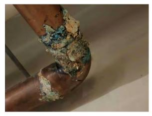
**Photo #99** Close-up of excessive electrolysis corrosion that may lead to leaking pipe soon.
