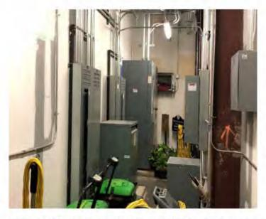
Main Switchgear Room. Recommend Eliminating Stored Material
