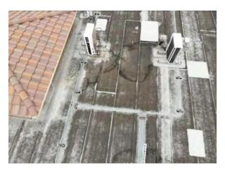
**Photo #37** View of staining on the modified bitumen roof.
