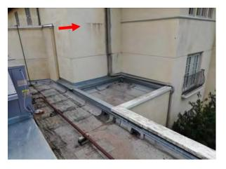
Photo #50 View of staining on stucco façade.
