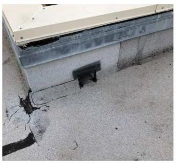
Scupper Opening On Interior Parapet Wall
