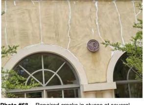
**Photo #68** Repaired cracks in stucco at several locations.
