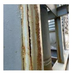
**Photo #61** Cooling tower structure shows deterioration and cracking. Close up of structural member.
