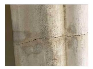
**Photo #64** Typical cracking stucco at several locations.
