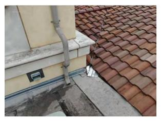
**Photo #45** View of downspout with no splash block.
