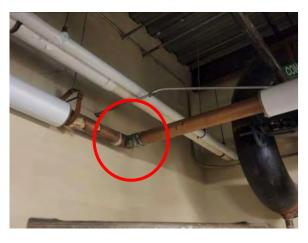
**Photo #98** Electrolysis corrosion on copper water distribution piping.
