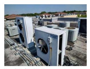
**Photo #113** Older DX split system condensing units on the roof.
