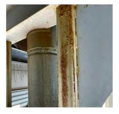
**Photo #60** Cooling tower structure shows deterioration.
