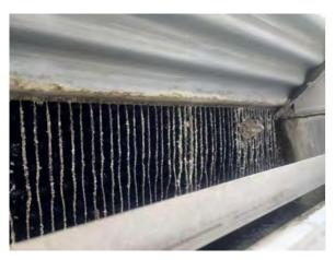
**Photo #94** Excessive scale built-up on cooling tower fill and louvers. Note: "Cooling Tower Fill" is media (plastic typically) used to exchange heat between the entering and leaving cooling tower water with the air being blown across it
