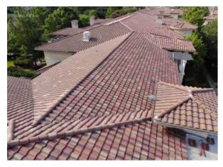
Photo #20 Close view of concrete tile roof.
