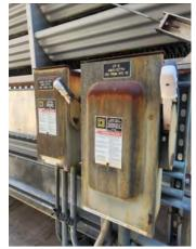
**Photo #95** Original to construction electrical disconnect for cooling tower fan.
