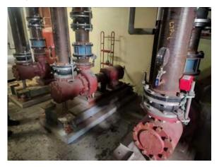
Photo #96 Cooling tower water pumps.
